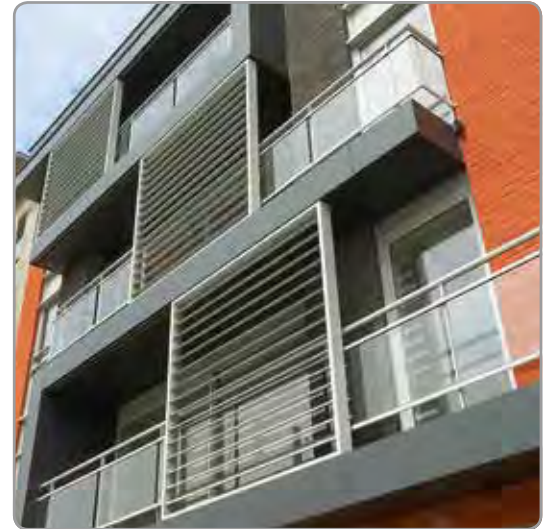
Loggia®, apartments, Kortrijk (BE)
