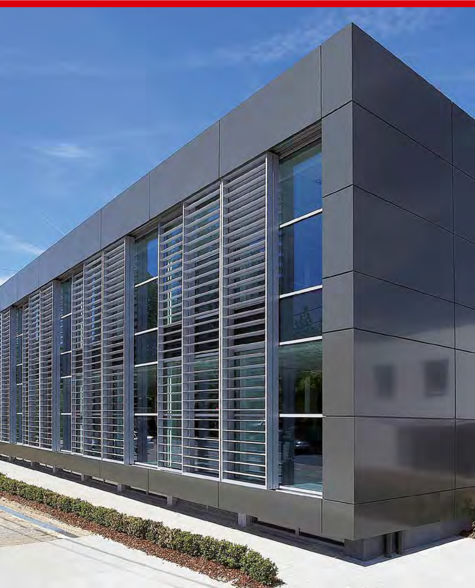
Loggia® 130 with Icarus® 125, TMWV Offices, Asse (BE)
